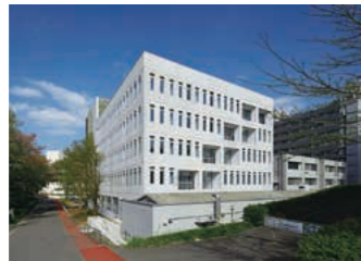
元素戦略研究センター (2015年、意匠：村田涼、安田幸一／構造：竹内徹) Materials Research Center for Element Strategy (2015, design by Ryo Murata, Koichi Yasuda / structure by Toru Takeuchi)
